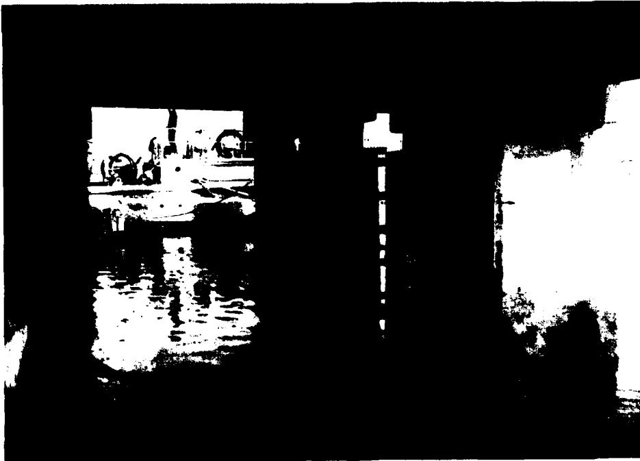
Photo V.10 WWF installed on piles A3, form installed on Piles B3 and completed repair on piles C3
