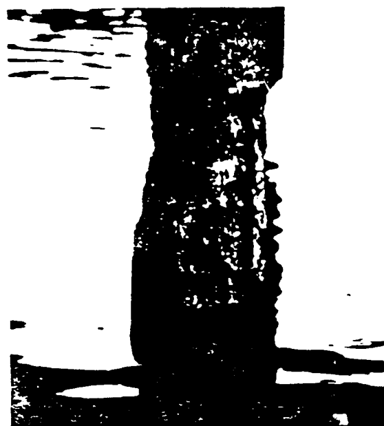
Typical condition where Types V or VI jacket should be used.
