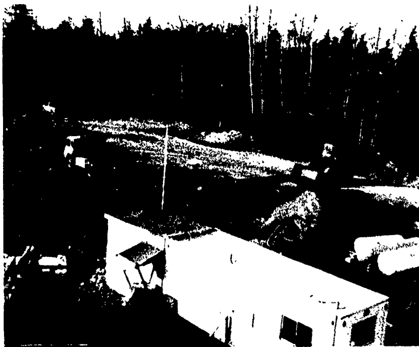
Winterization. Steel pipe arranged for the sand stockpile. The building is the contractor quality control laboratory.
