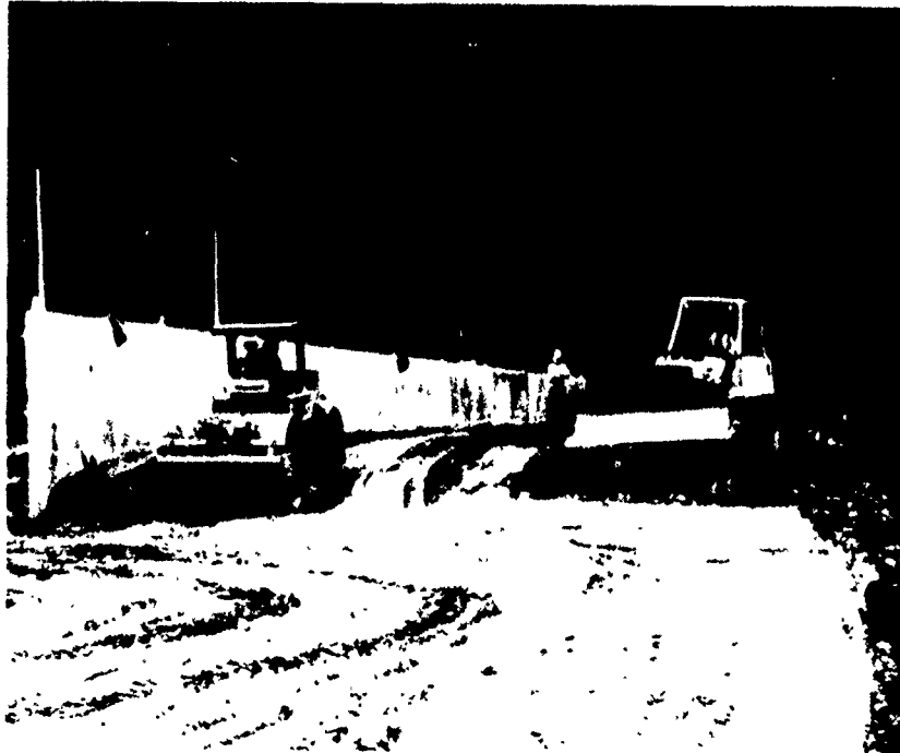
Backfill and compaction during dam raising. Thin strip either side of CIP wall was compacted with hand-operated tamper.
