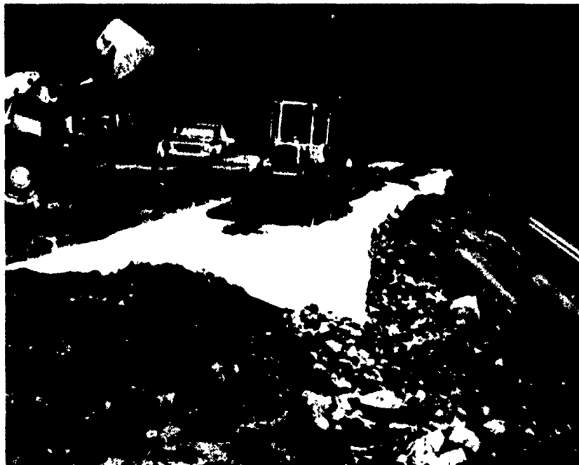
Geotextile placement on lowered dam work platform. 6" of base course material over fabric.
