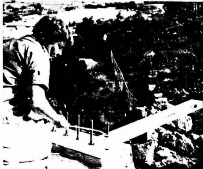
Fig. 8 Simple cantilever test assembly for flexure tests of weathering acrylic specimens
