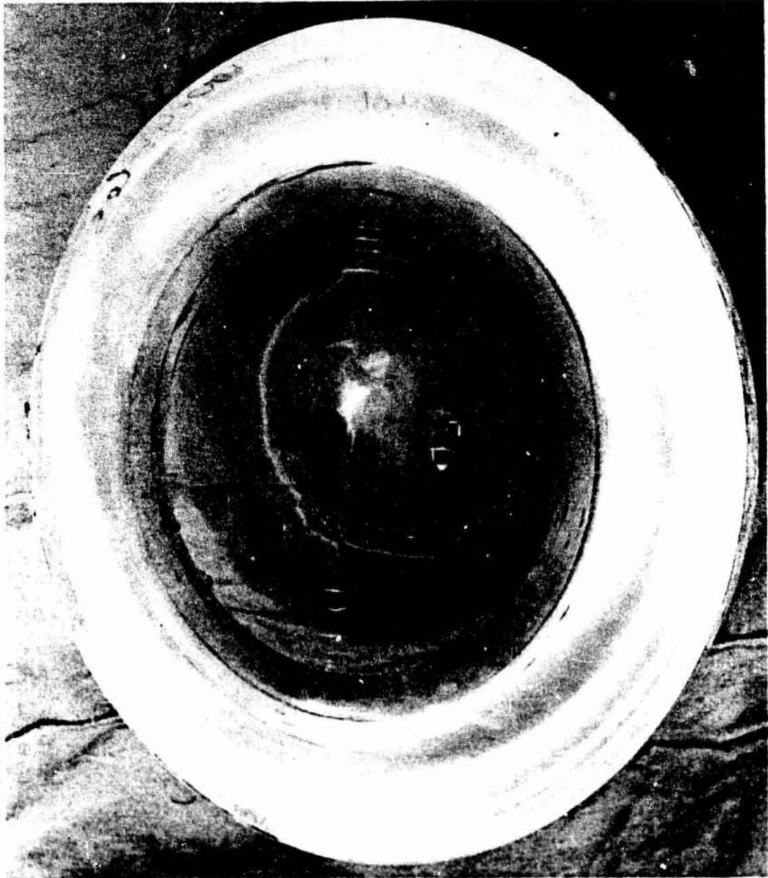
B. BOTTOM VIEW; NOTE FEW CIRCUMFERENTIAL CRACKS IN BEARING SURFACE NEAR INSIDE DIAMETER.
