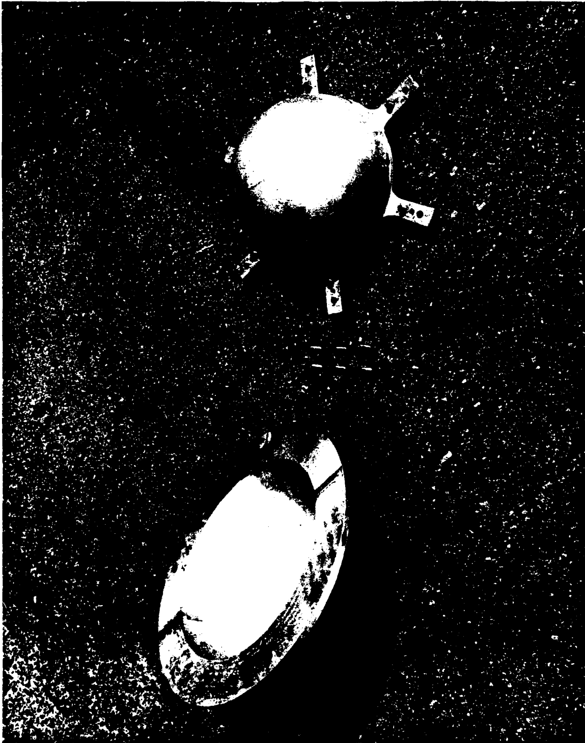
Figure A-4. Concrete hemisphere mold, disassembled.
