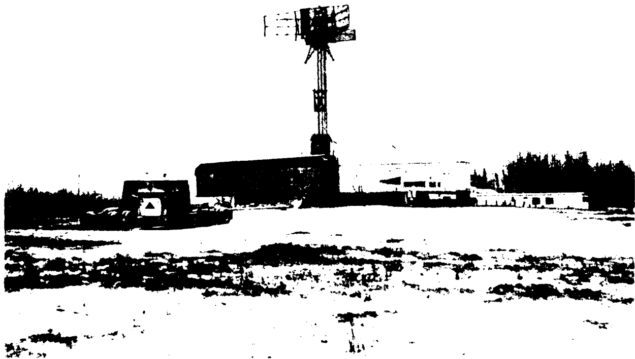
Figure E-49. Phase One at Woking. Equipment on site
