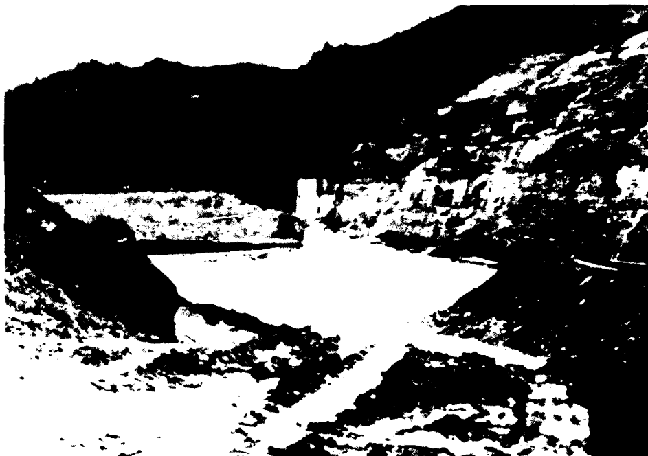
Figure 8. Breach of R. D. Bailey cofferdam looking upstream
