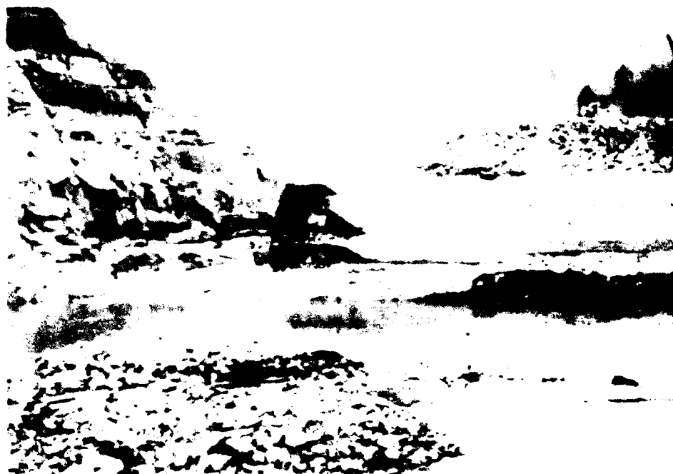
Figure 9. Breach of R. D. Bailey cofferdam looking downstream
