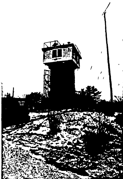
Left: Building #32 (Maritime Tower), currently being restored.
