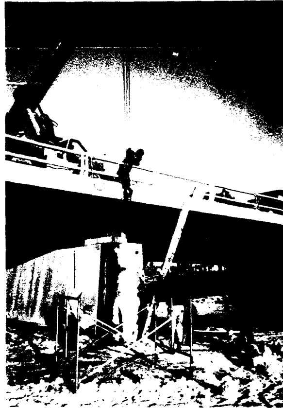
Figure 3. Installation of the ice force panel in December 1989.
