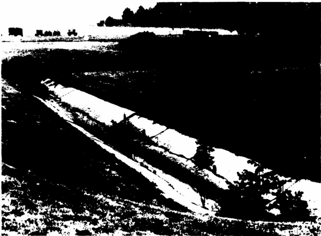
Figure 6. Drainage Ditch to Storm Water Holding Pond.
