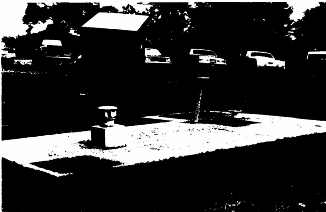
Figure 8. Oil/Water Separator, Site 13.
