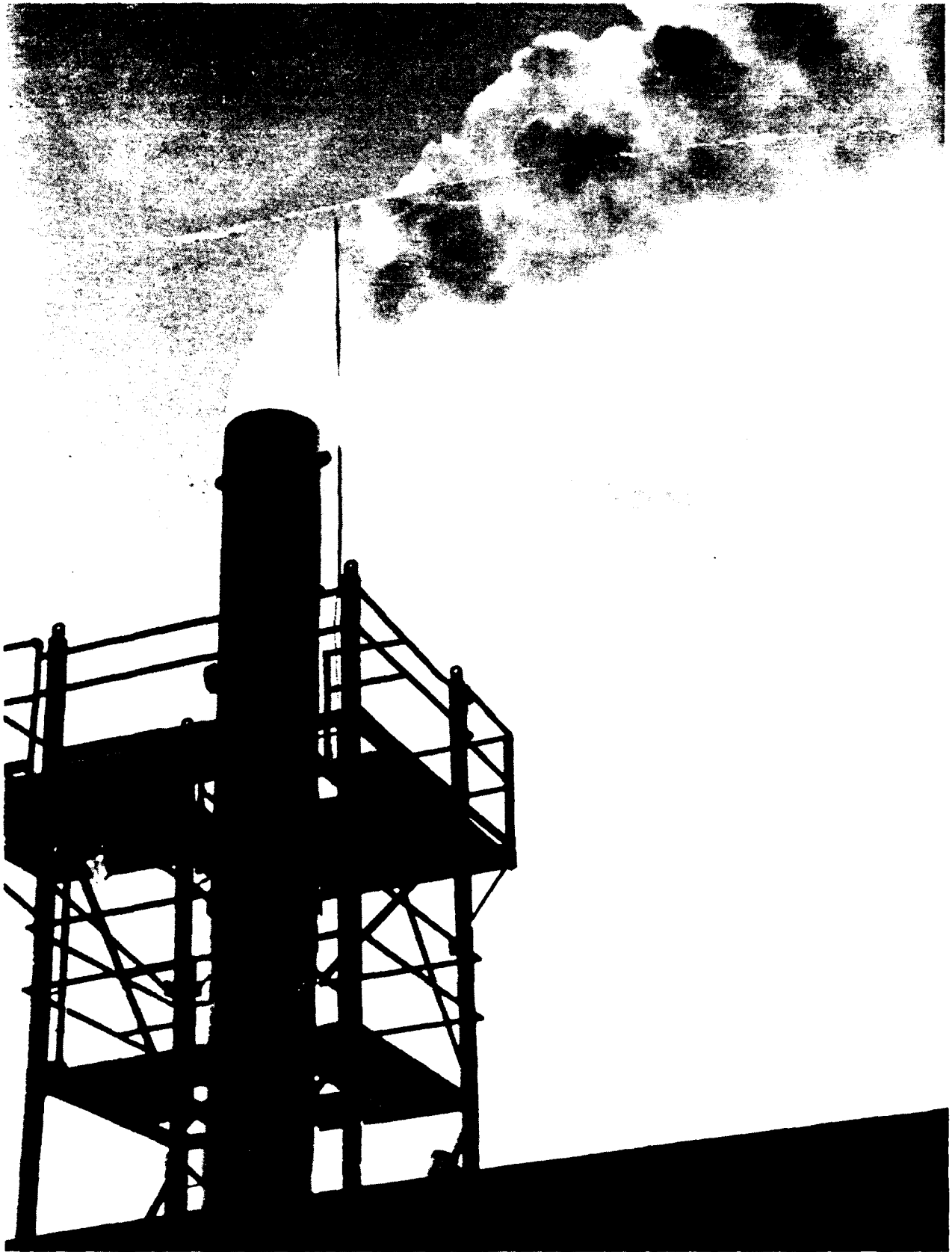
Figure 12. View of Incinerator Stack.
