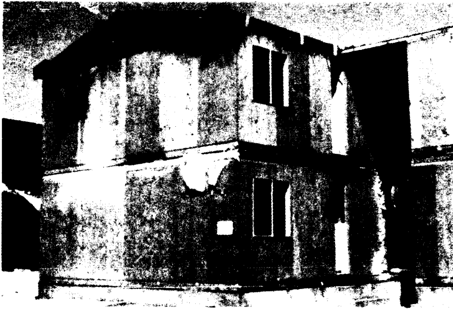
Figure A5. Completed assembly of modules.
