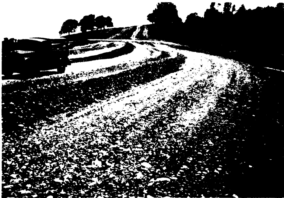
Figure 21. Placement of Zone 1 upstream shell, looking southwest from sta 421+50 to right abutment (FOL-528)
