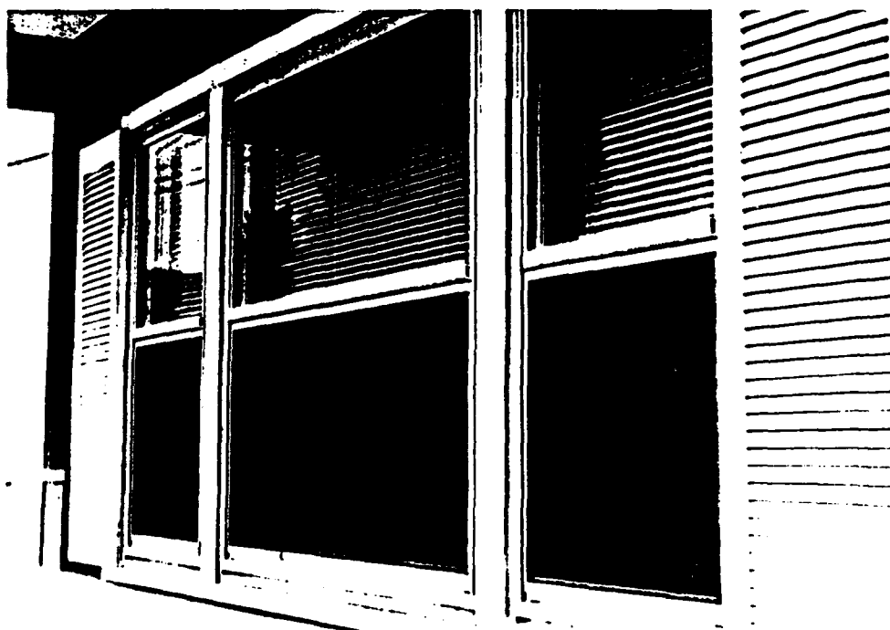
Figure 3-6. Typical Acoustical Windows in Place.
