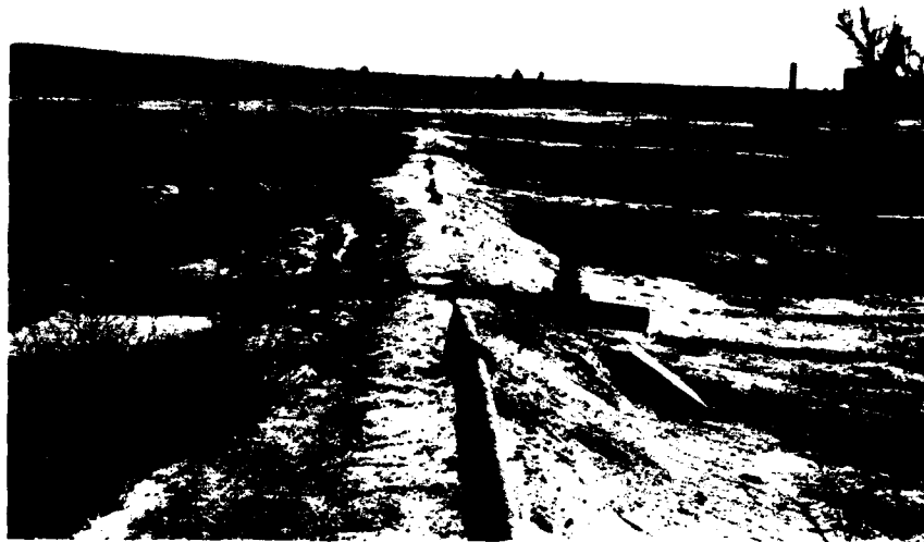
Figure 3. Inlet Pipes to the WWTP Sludge Drying Beds. Grab sample for "hot spot" sample taken below end of pipe.
