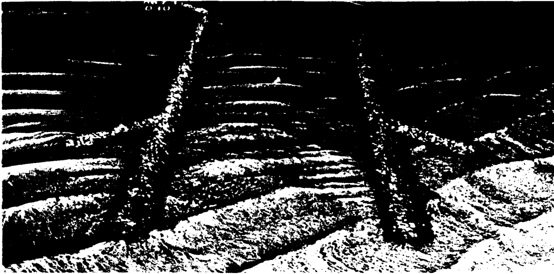
Figure 11. Optimum location of jetty spurs for prevention of shoaling at Siuslaw River, Oregon
