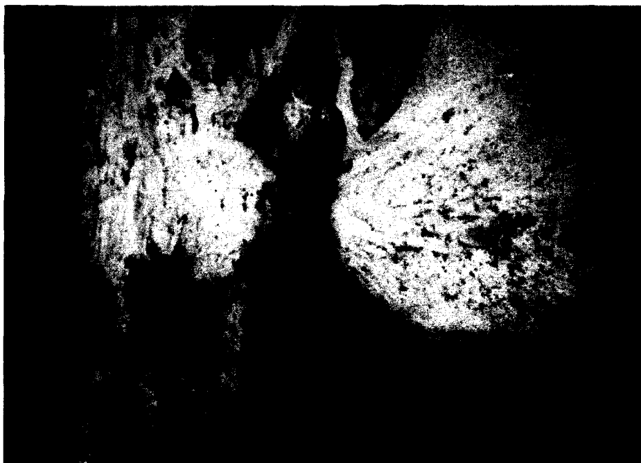
a. Fine sand "fan" below piping cavity (top) in bank
