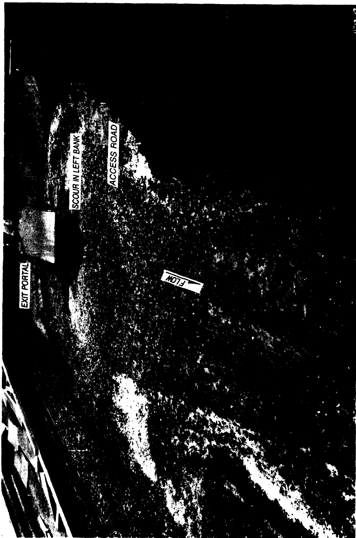
Photo 16. Scour, type 4 design energy dissipator/preformed scour; discharge 8,000; pool el 2580; 1 hr (prototype)
