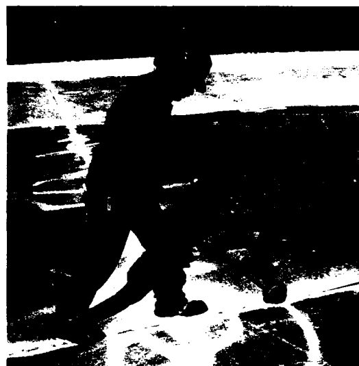
Installing a backer rod to maintain the proper shape factor in the joint.
