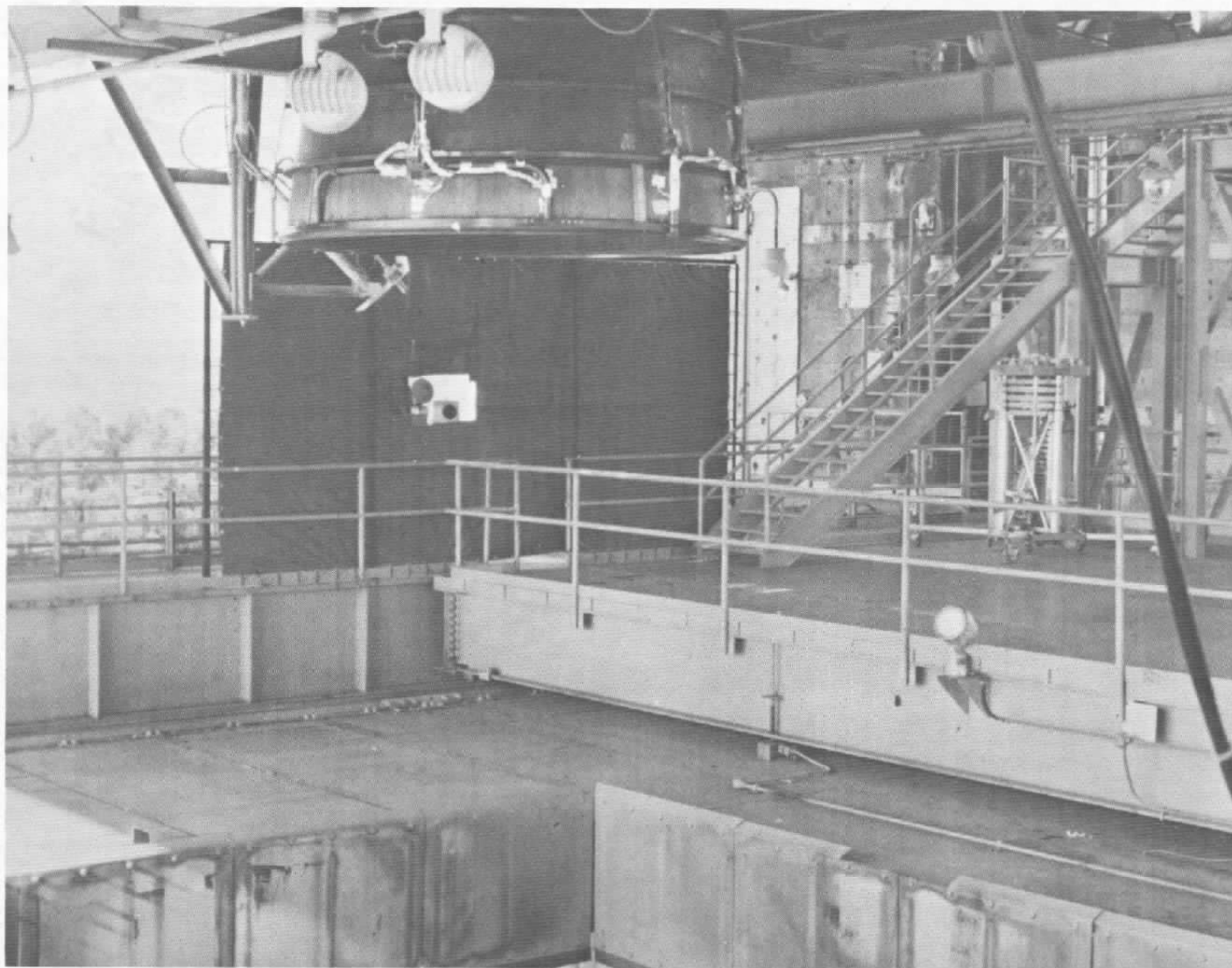
Figure 22. Photograph of Level 10 area.
