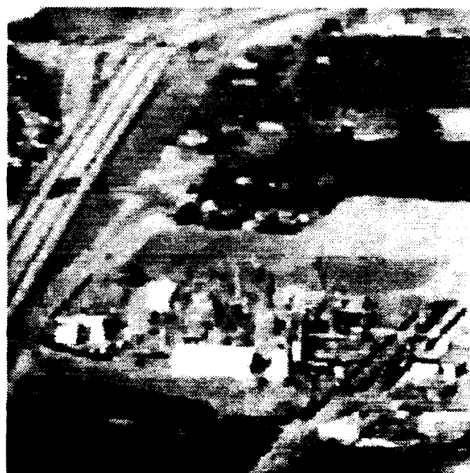
c) Restoration of "b"
