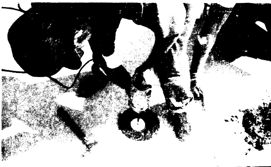
Figure 14. Staggered Anchoring Fasteners on Membrane B.
