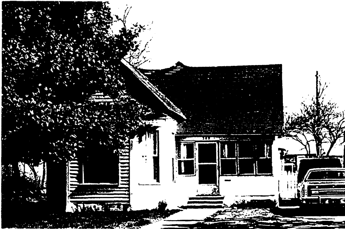
Figure C-15. NLU-83-125, Victorian L-Shaped Cottage with Decorative Peak on Roof.
