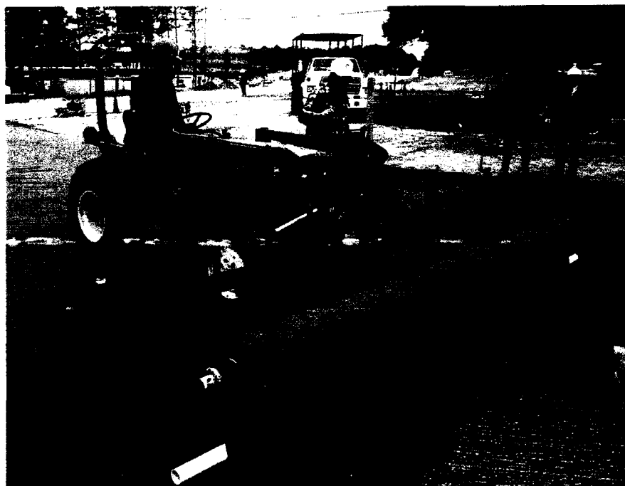
Above: A small tractor was used to place the geotextile at Ft Jackson. Top right: Applying cover aggregate on the asphalt-rubber at Ft Sill. Bottom right: Placing the asphalt concrete overlay at Ft Jackson.
