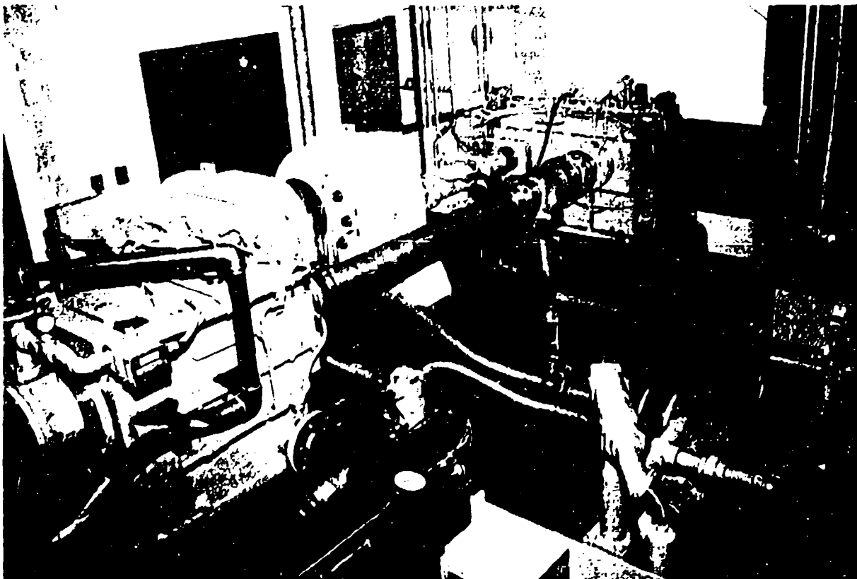
Figure 108. ART Gearbox Installation
