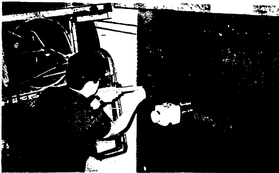
Figure 4.10 Measuring the out-of-flatness of a plate girder web.
