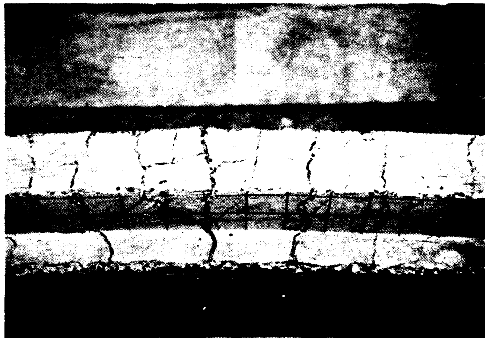
Figure B20. Test Beam #1 - #5 Rebar, Flexural Cracks
