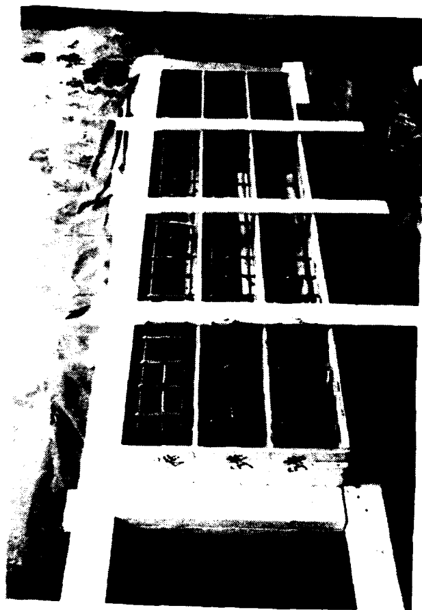
Figure B11. Small Form and Rebar Cages
