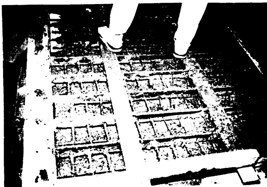
Figure B13. Placement of Concrete
