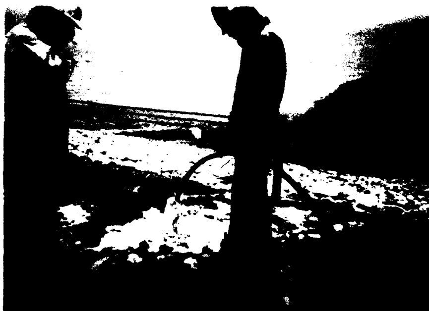
(Photo 12) Washing out a hole prior to testing and grouting
