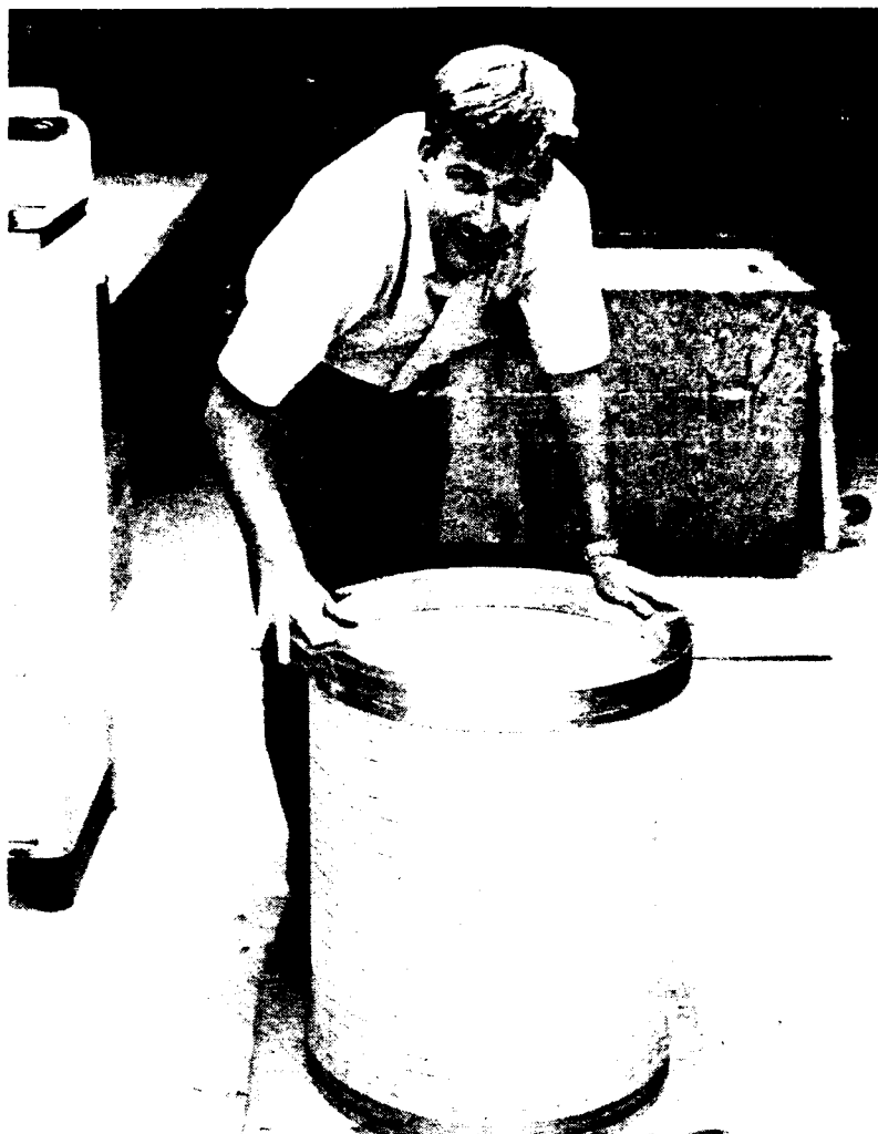
Figure 26. Cylinder A with Mod 1 aluminum end cap rings marked up for ultrasonic NDT.
