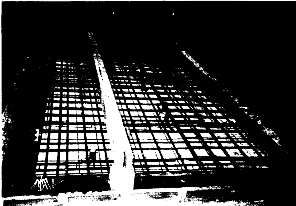
Figure 6. Form and reinforcing steel ready to pour
