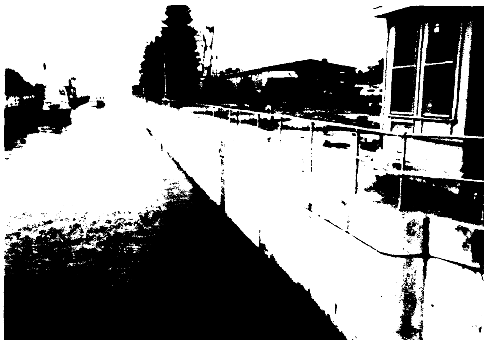
Figure 22. Rehabed lock chamber returned to operation
