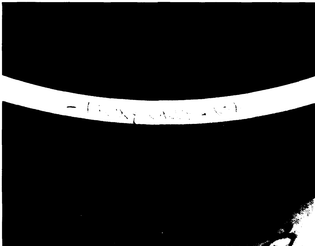
Figure 22. Crack-free bearing surface at the bottom end of the Test Configuration B cylinder.
