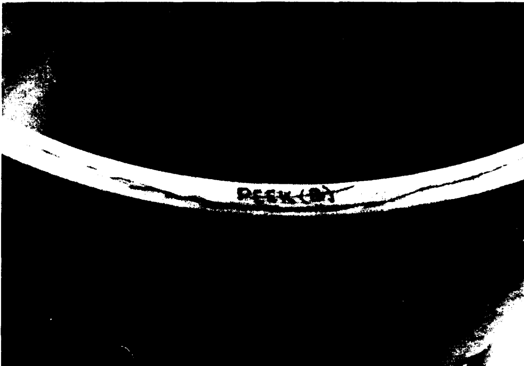
Figure 21. Bearing surface cracks at the top end of the Test Configuration B cylinder.
