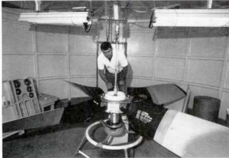
Figure 27. Balancing C-130 Aircraft Propellers. This is a depot maintenance activity performed at the Warner Robins Air Logistics Center, Georgia.
