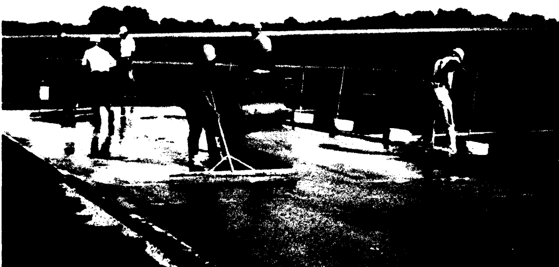
Figure 23. Removing excess slurry grout from surface
