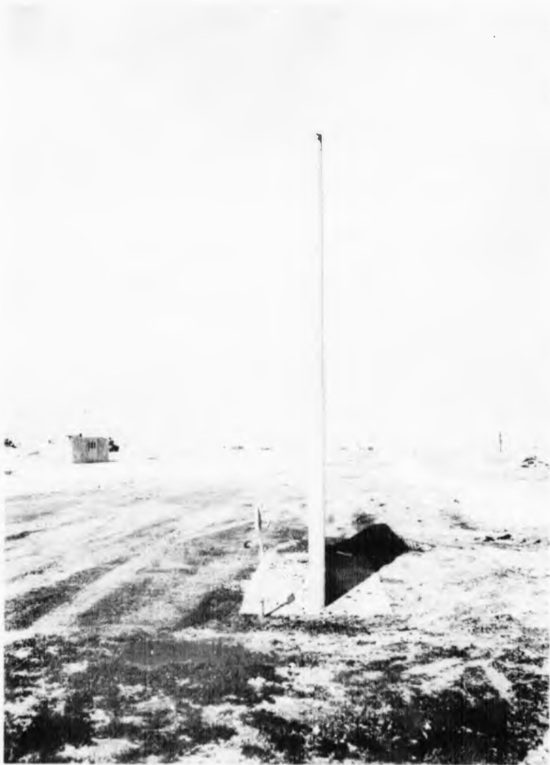
Fig. 3.6 Test Easy, Station 37b; End View of Pylon toward Zero
