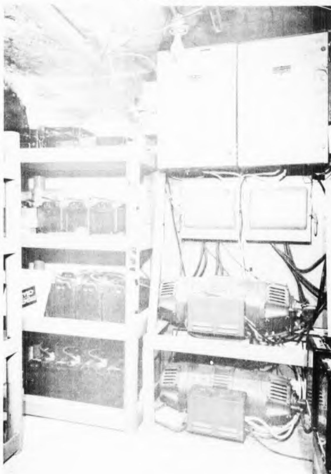
Figure 1. Cabinet of Four 8000 Watt Huz Converter
