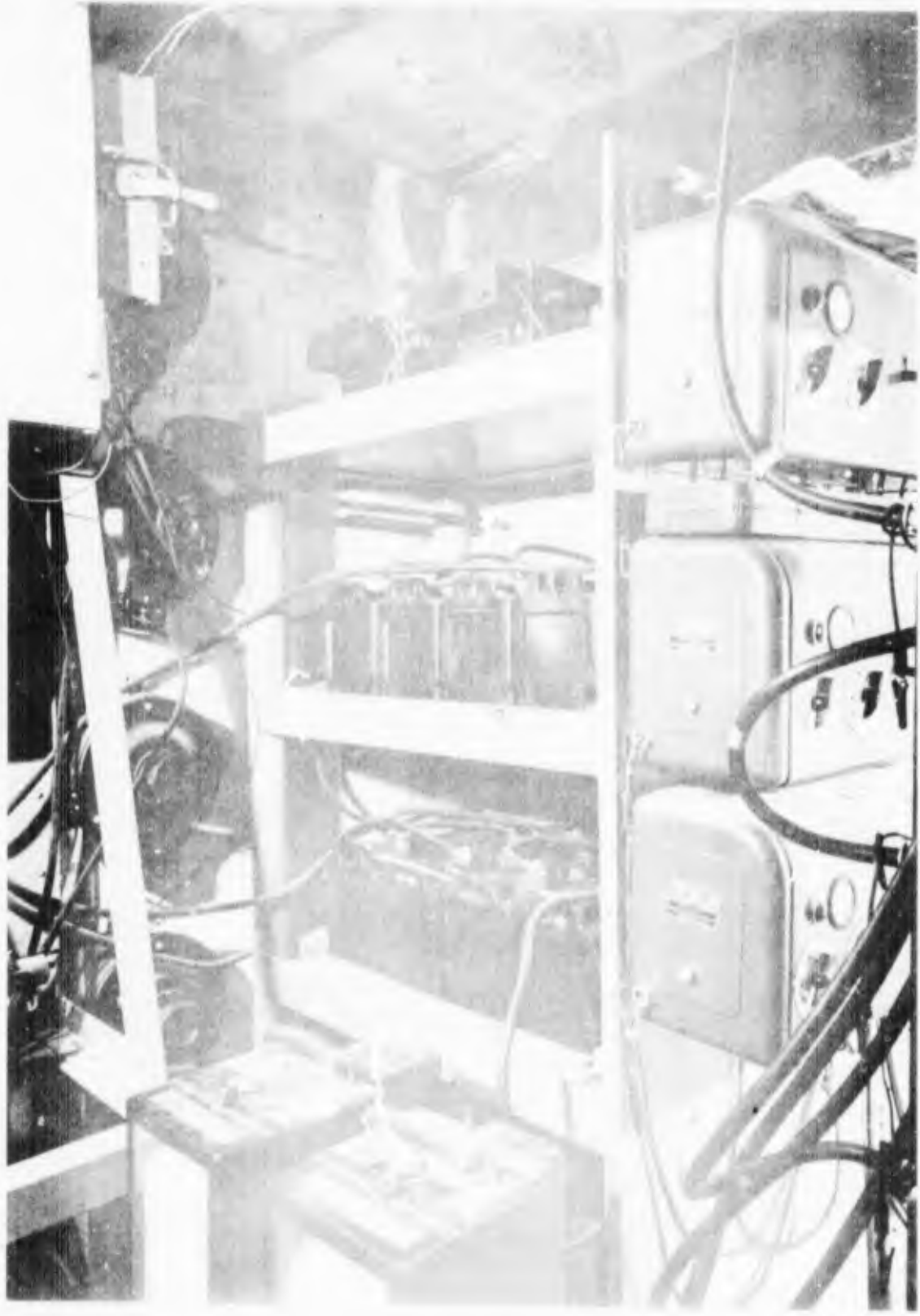
Fig. 14. CONTROL ROOM (PARTIAL) OF THE "SAGE" SYSTEM
