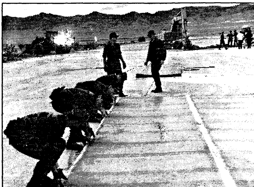
Folded fiberglass mats being unfolded and installed.
