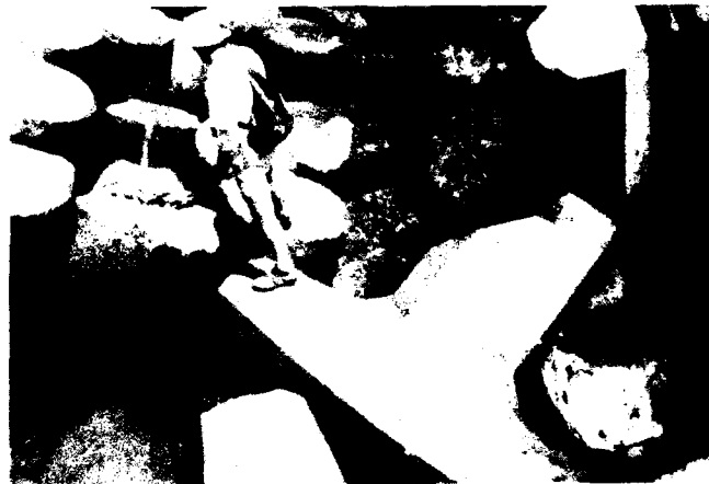
Figure 7. Tribar failure at central node
