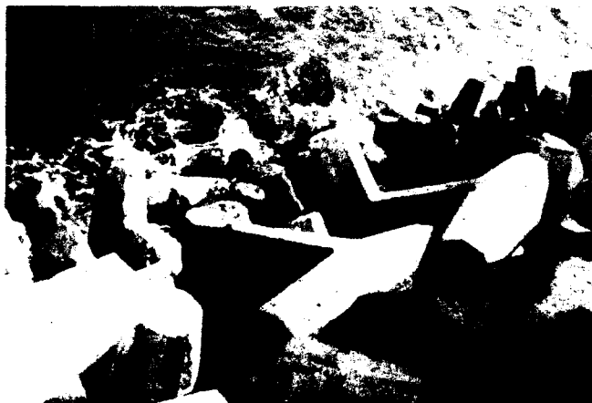
Figure 6. Dolos with fluke section sheared off
