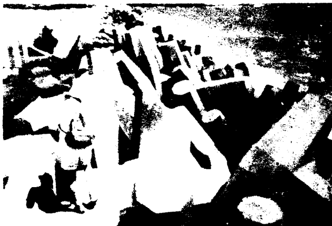
Figure 4. Typical torsion break of dolos shank
