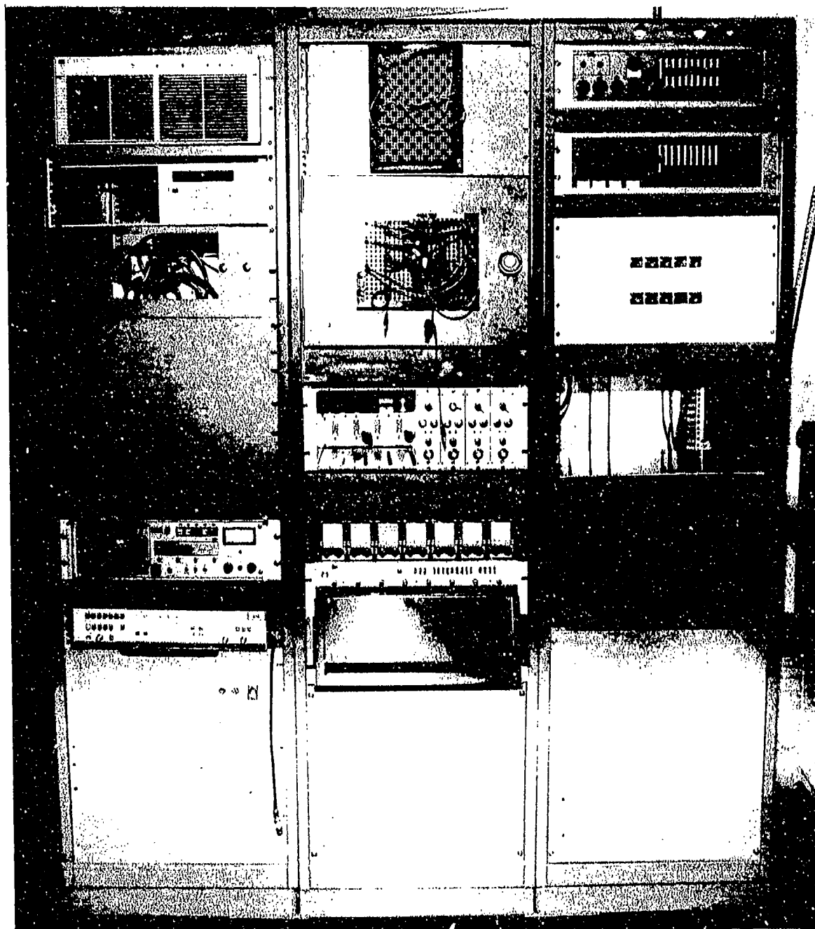
Figure 13. The front side of instrument racks in the control room.
