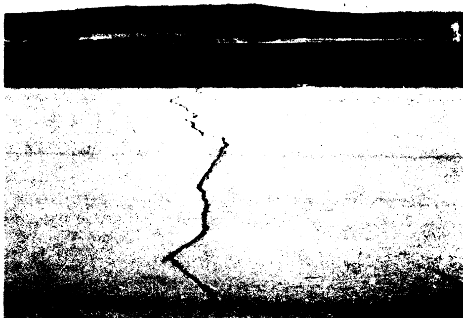
Figure 7. Typical transverse crack in Item 4 (Taxiway 1 E/W)
