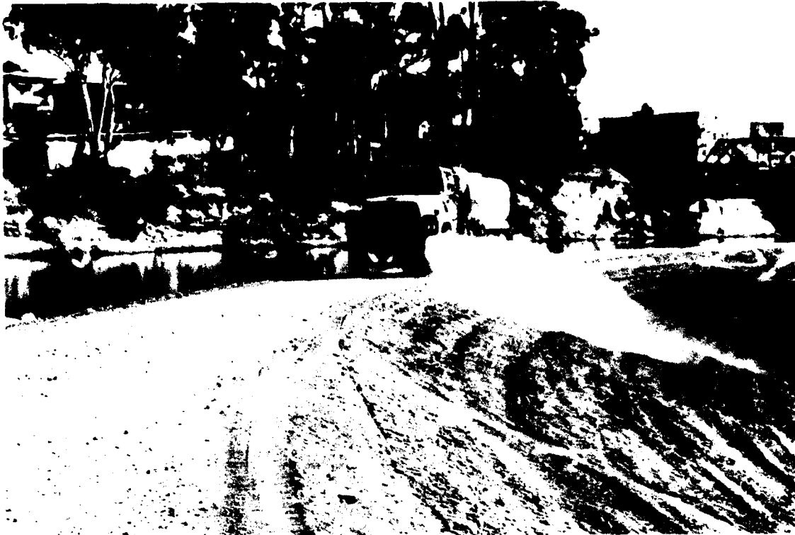
a. Water truck, watering slope during levee reconstruction
