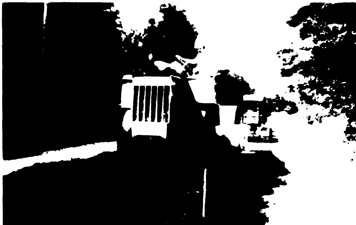
Figure 8. Compacting the tire chips with the vibratory roller.
