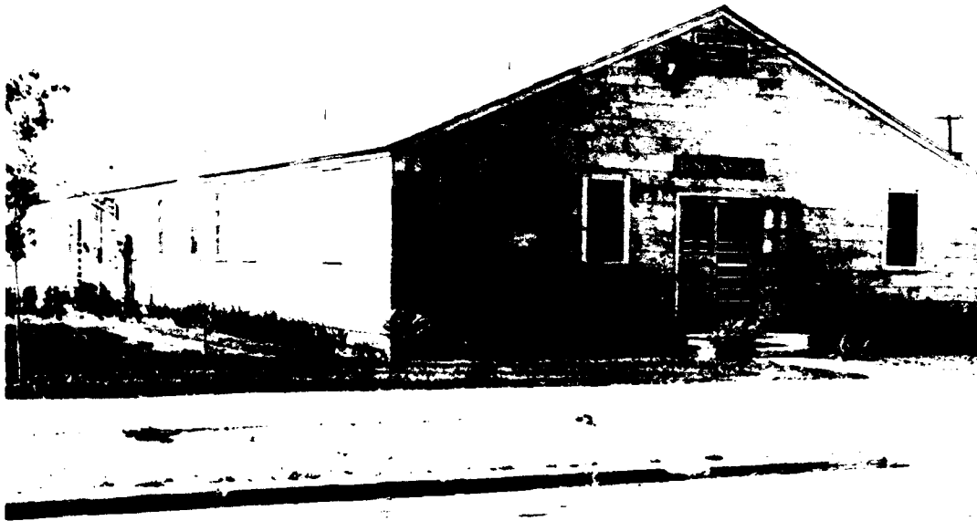
FIGURE 24.—Typical industrial dispensary.
