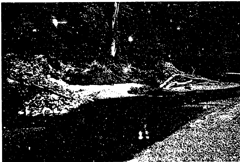
Plate 8 : Whole tree and smaller timbers on bendway weirs. Harland Creek (23)
