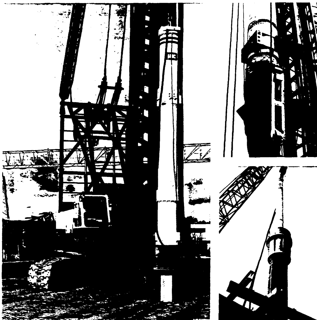
Figure F-2 Underwater Pile Driver (Figure from IHC Hydrohammer literature)
