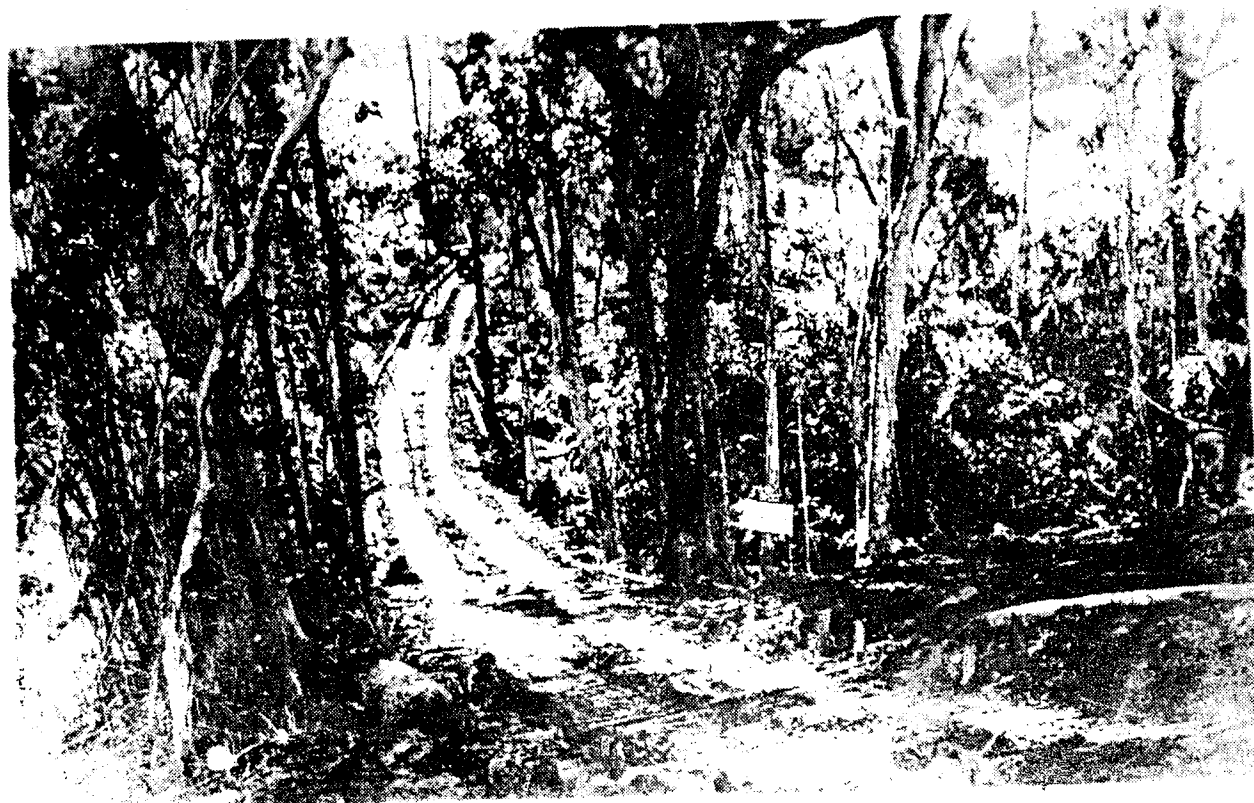
TERREL BRIDGE (NOTE CORDUROY ROAD )
