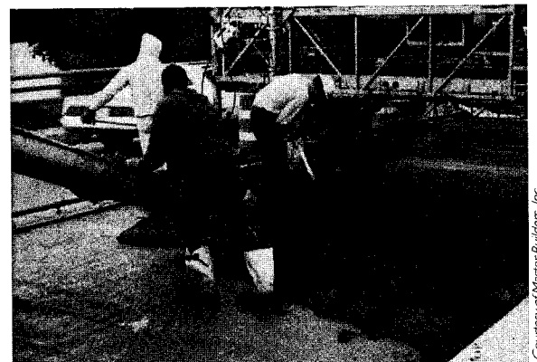
Placement of a HPC silica-fume concrete bridge deck overlay by Ohio Department of Transportation. This use of silica-fume concrete takes advantage of the low permeability of the concrete to slow the rate of chloride ingress.
