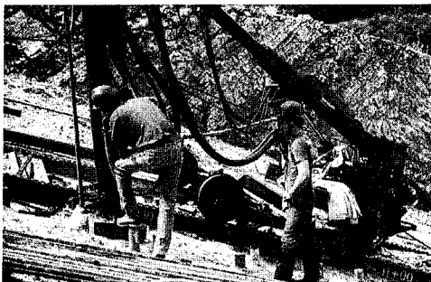
Photo courtesy Hayward Baker Inc.
