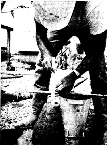
A worker performs a slump test.
