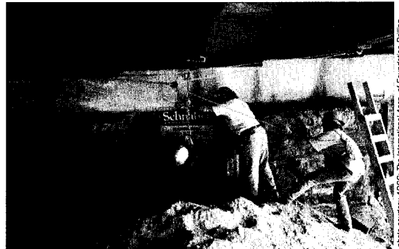
Prior to starting excavation work under the I-285 overpass in Atlanta, Ga., crew members of the Schnabel Foundation Company practiced confined space rescues using lifelines and pulleys.
