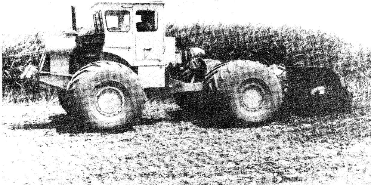
Figure 7. GEMCO vehicle with Dondi ditcher being lowered into position for trenching
