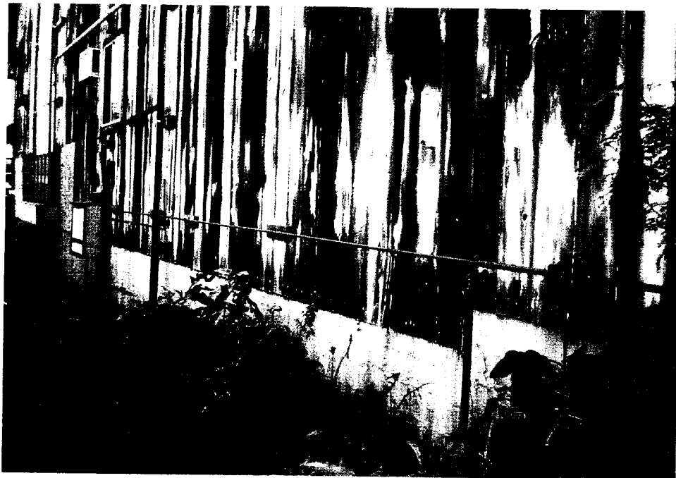
4. View showing peeling paint on side of Armory Building.
