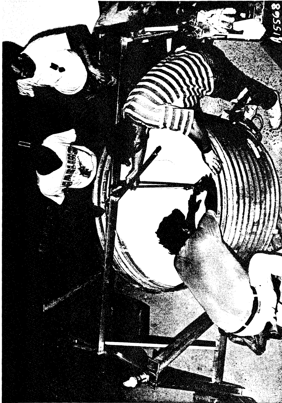
Figure 2-7. Photograph of personnel placing gages in the target.
