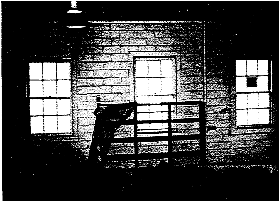
BUILDING NO. 337: Interior. (Looking South) Date of Photograph: 27 August 1982
