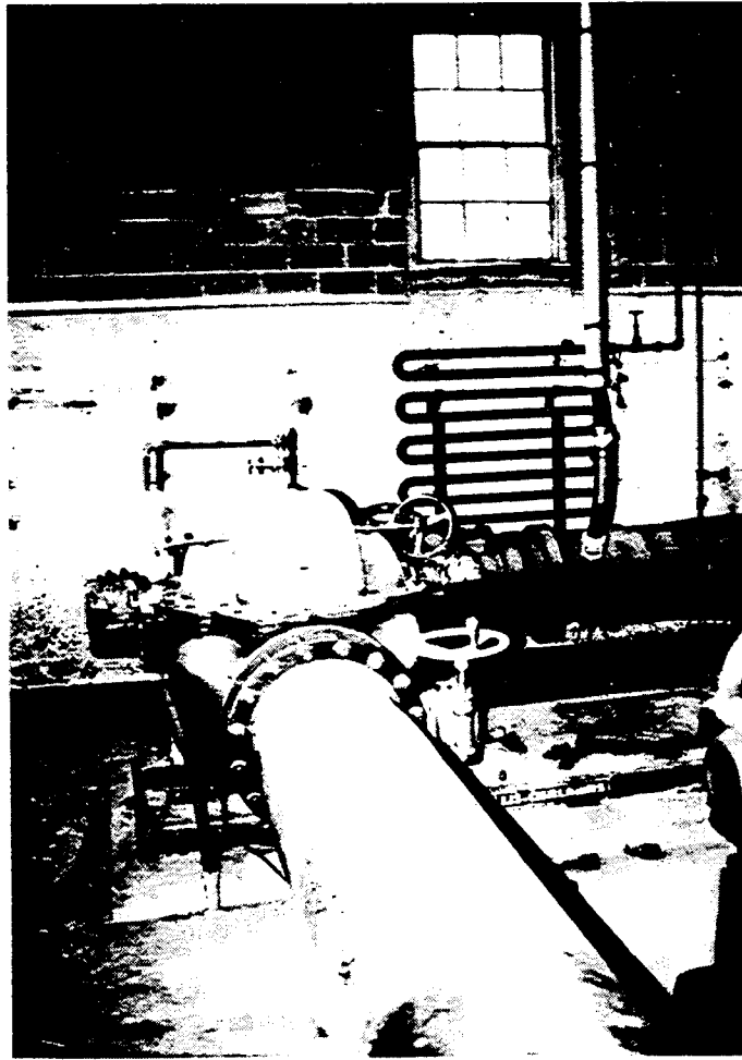
BUILDING NO. 326: General View. Circulating Pump. Date of Photograph: 27 August 1982
