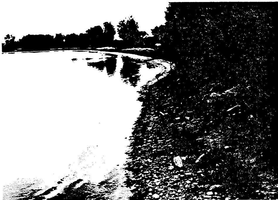
LOWER DERBY LAKE: Dike and Riprap. (Looking South) Date of Photograph: 26 August 1982
