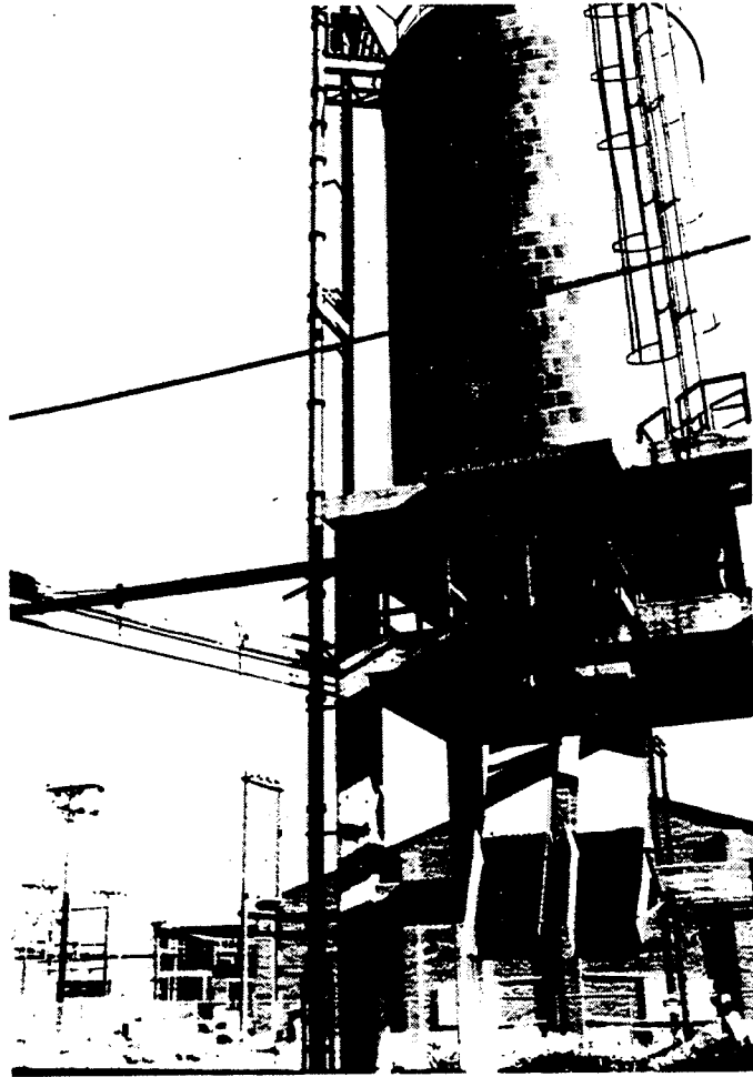
BUILDING NO. 323: Ash Silo and Air Wash Date of Photograph: 31 August 1982
