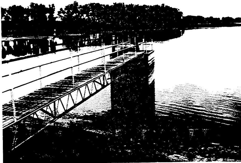
LOWER DERBY LAKE: Sluice Gate Structure Date of Photograph: 26 August 1982
