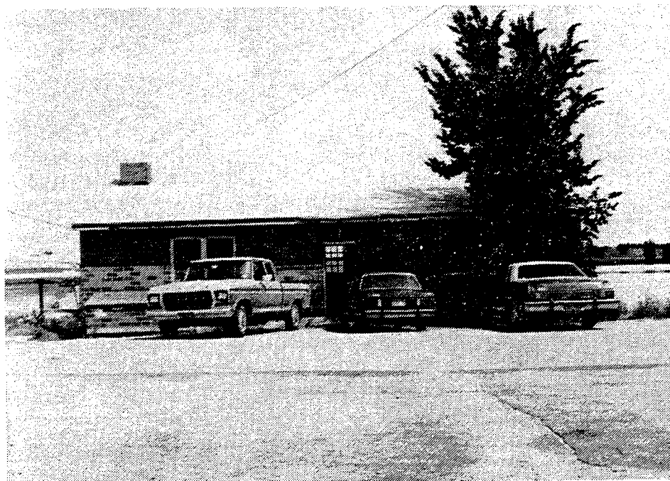
BUILDING NO. 371: West Elevation Date of Photograph: 26 August 1982
