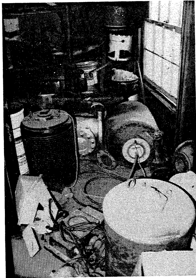
BUILDING NO. 322: Interior. Miscellaneous Equipment Date of Photograph: 7 September 1982
