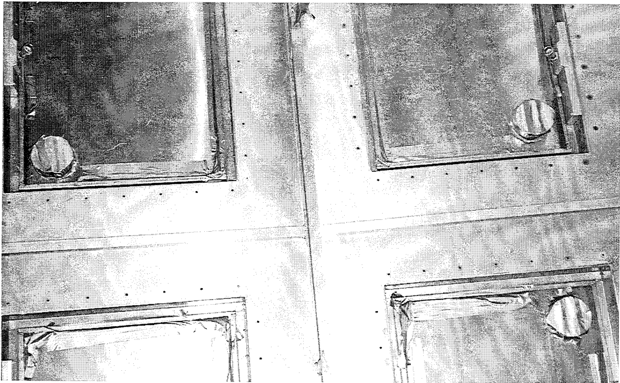
Figure 9. New roof vent covers viewed from inside of the MKT.
